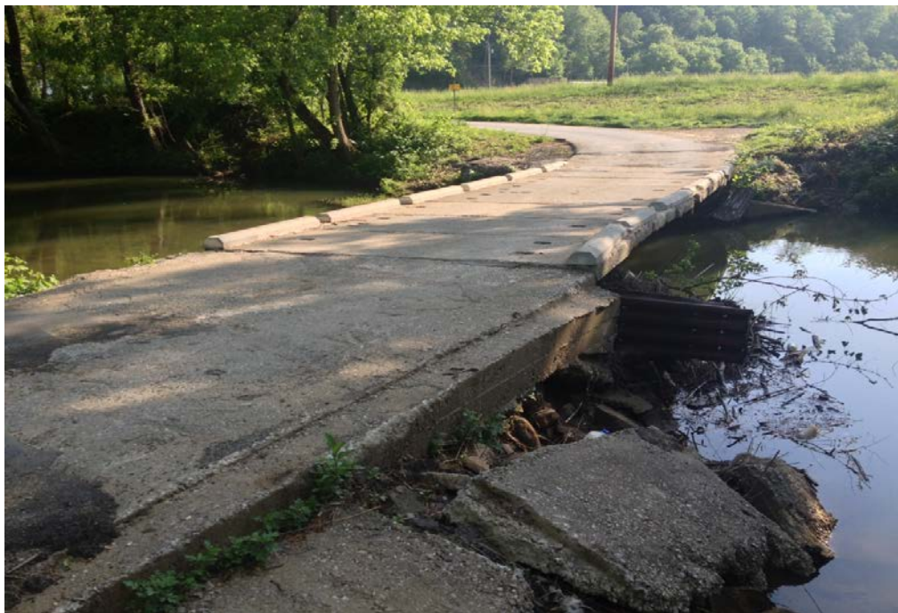
Looking north-east at bridge
