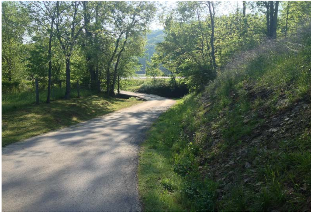
Approaching the bridge from the south-west, looking north-east
